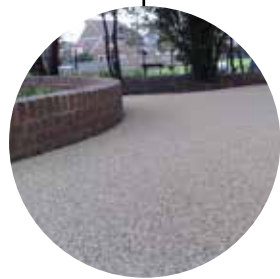
Resin bound gravel surface
